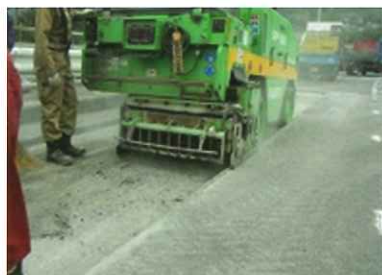
① 舗装の切削
